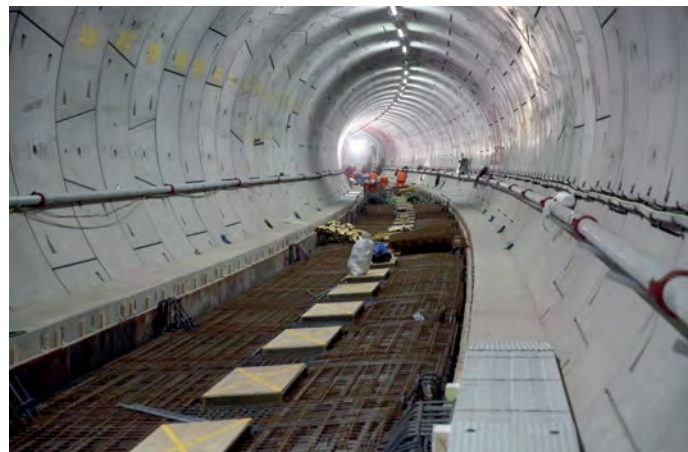
Floating track slab preparation beneath Soho, between Tottenham Court Road and Bond Street. The blocks will 'bookend' the sprung track.
