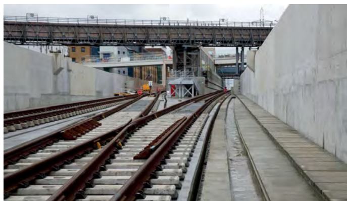
Track and switches installed west of Custom House station where the route climbs eastwards from Victoria Dock portal.
