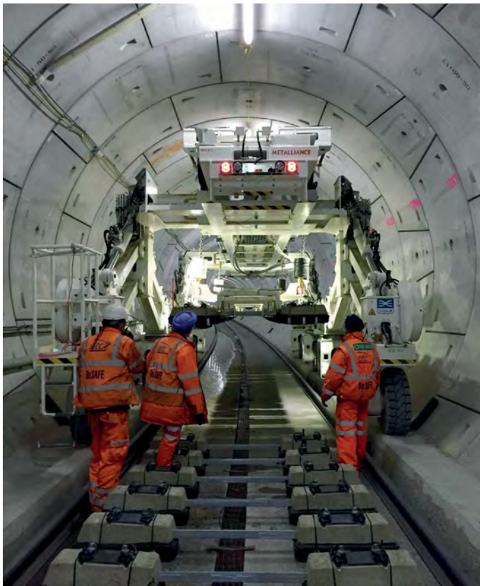
Multi-purpose gantry lifting sleepers into place in Thames Tunnel in November 2015. All photographs courtesy of Crossrail
