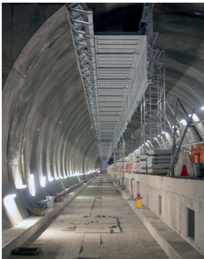
Bond Street station platform in February 2016, with brackets in place for platform edge screens and ducts above the track. Air extraction duct openings can be seen in the platform side.
