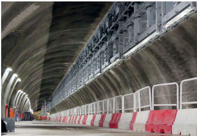
Bond Street station platform in January 2016 with brackets in place for platform edge screens.
